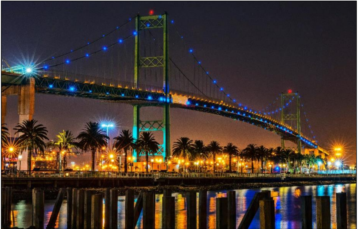
Vincent Thomas Bridge at Night, 1st Place
