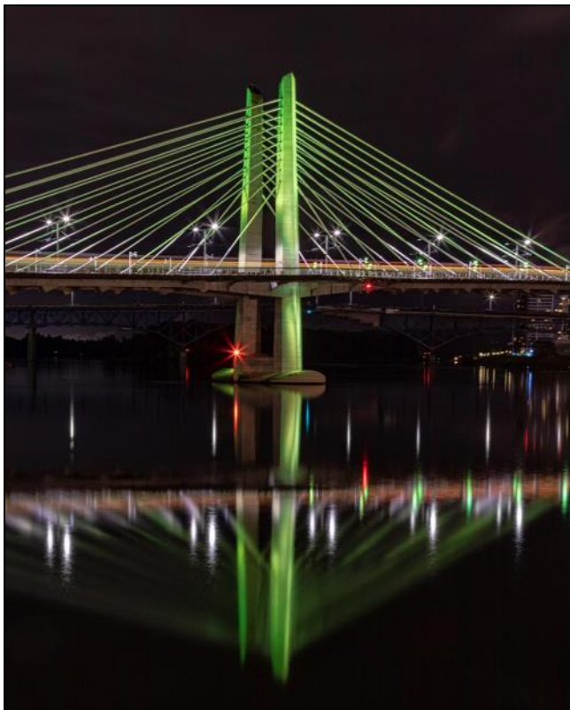
Portland Bridge - George Harper
